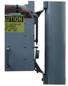
2. Remove the padlock and rotate the collar out of the way. Place handle over the exposed shaft and insert interlock pin. Switch is now operated like any manual switch.
