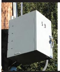
The MSO is available in a choice of powder-coated mild steel or stainless steel enclosures. All enclosures have the following features:
